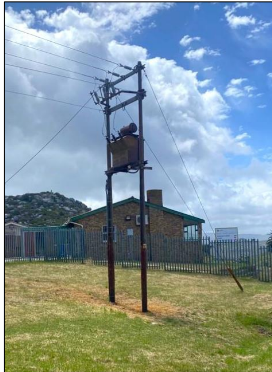
Figure 12. Potentially problematic electrical infrastructure, such as this H pole, is inspected on a regular basis.
